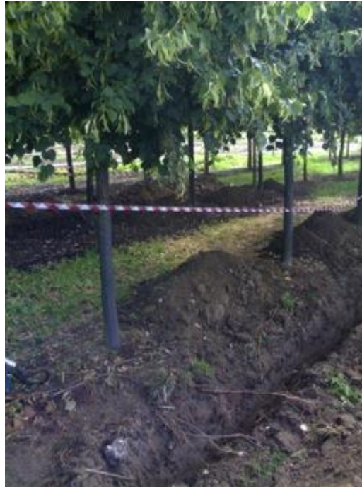
Trenching on 1 side of the tree - MD
